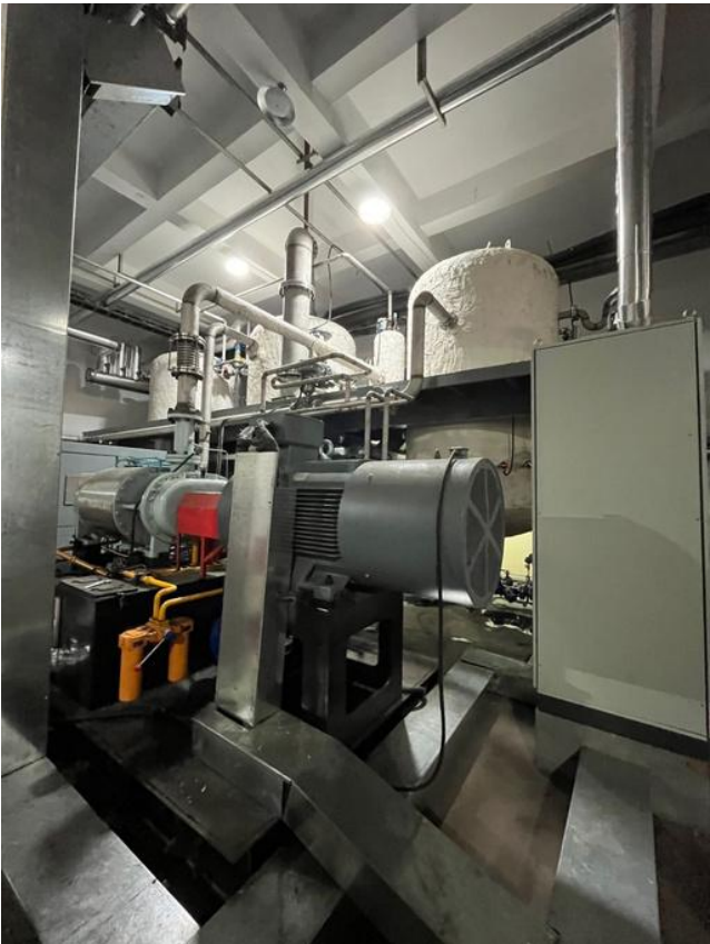
Heat pump in H&M Group China supplier
