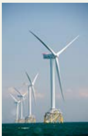
The Ormonde Offshore Windfarm, built in the Irish Sea, comprises of 30 RePower 5M wind turbines with the capacity of 150 megawatts and expected to produce around 500 gigawatt hours of electricity every year.
